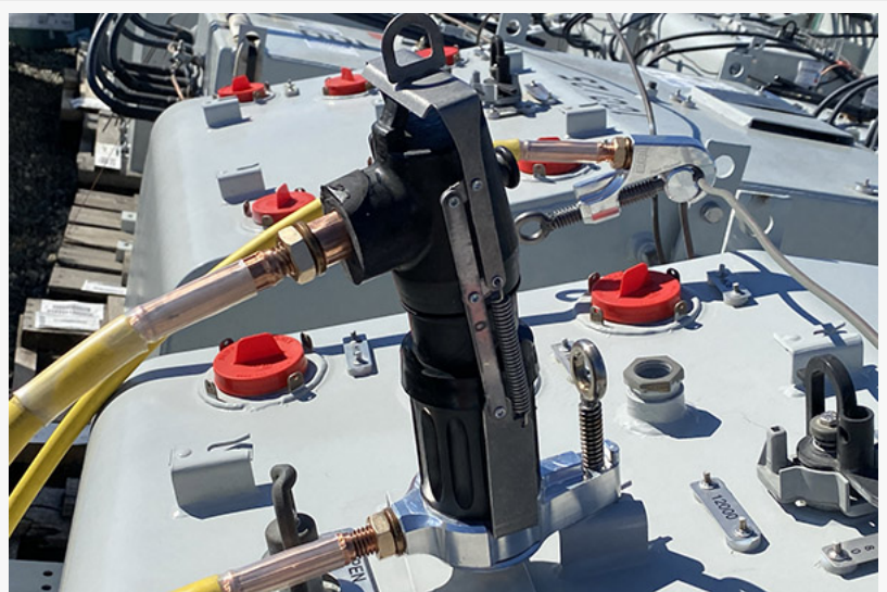
Grounded Bushing Well
