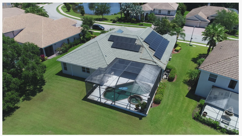
Mirasol Pool Heating
