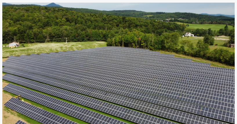
Lawrence Brook Solar project is providing low-cost renewable energy to Morrisville Water and Light customers
